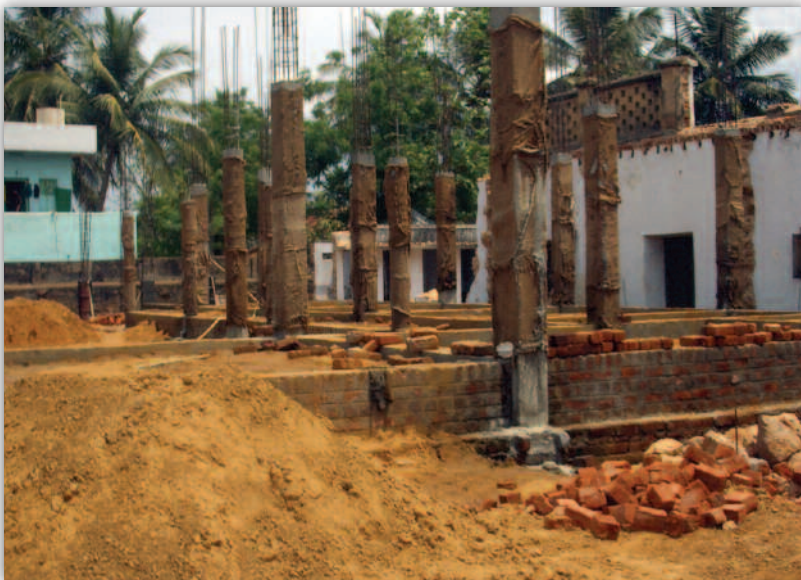
The girls hostel at Giffard Memorial Hospital under construction
