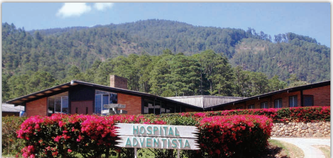
The entrance to Hospital Adventista de Valle de Angeles
