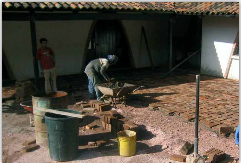
Refurbishing one of the buildings at HAVA
